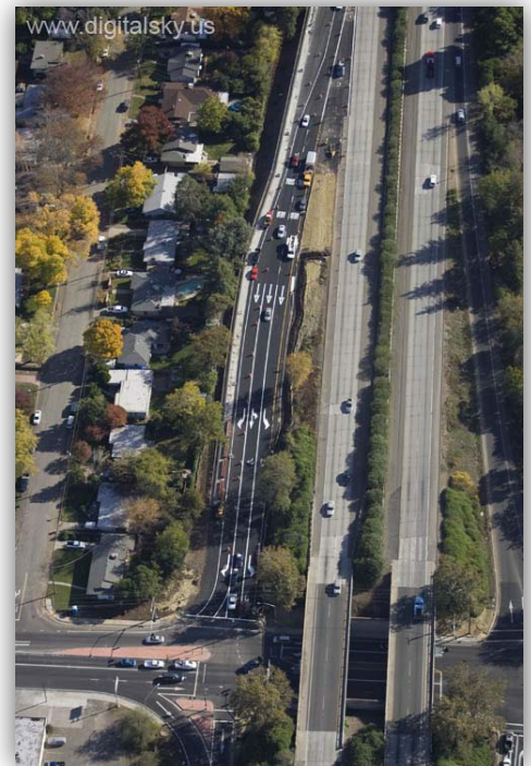
The new off-ramp at SR 99 & East First Avenue
