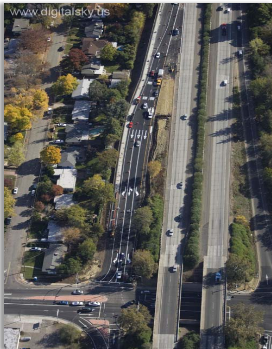
SR 99/East 1 st Ave Phase 1 Off-Ramp Improvement
